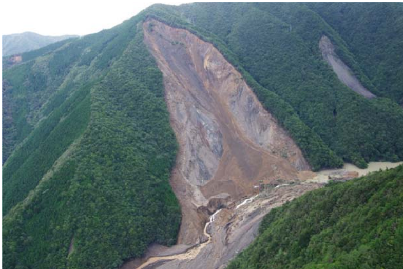
Deep seated landslide occurred in 2011
