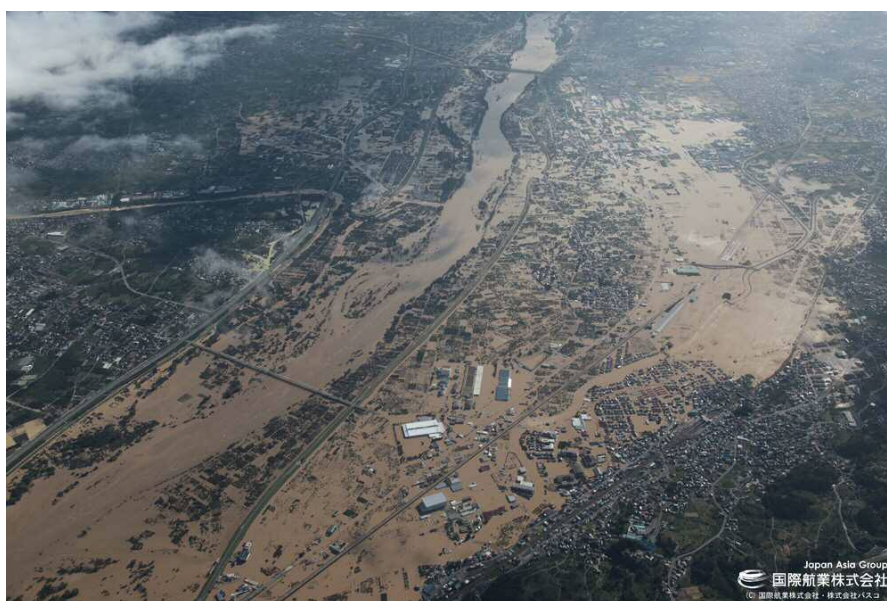
Flood disaster induced by typhoon 19th in October
