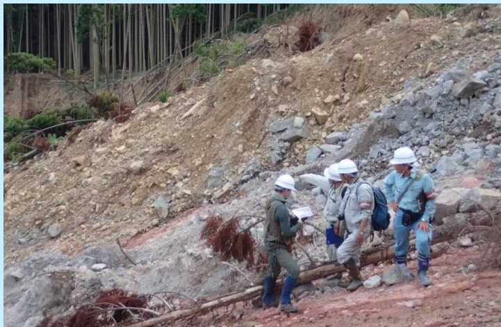
JSEG Investigation Team For Landslide disaster,2017
