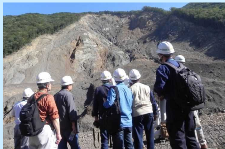
Large landslide, south of Kyoto
