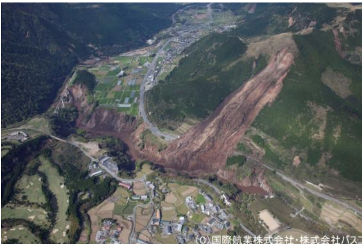
Fig. 8 Large collapse on the steep slope of near the somma of Volcano Aso (View from point A in the Fig. 7)
